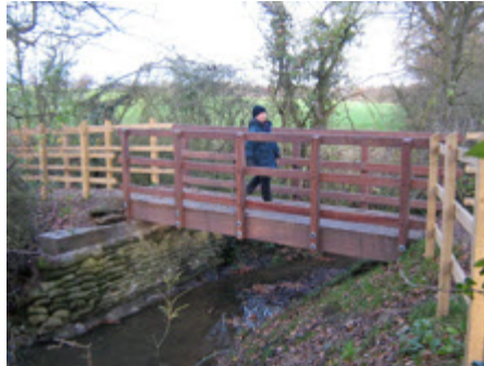
2009: the new footbridge
