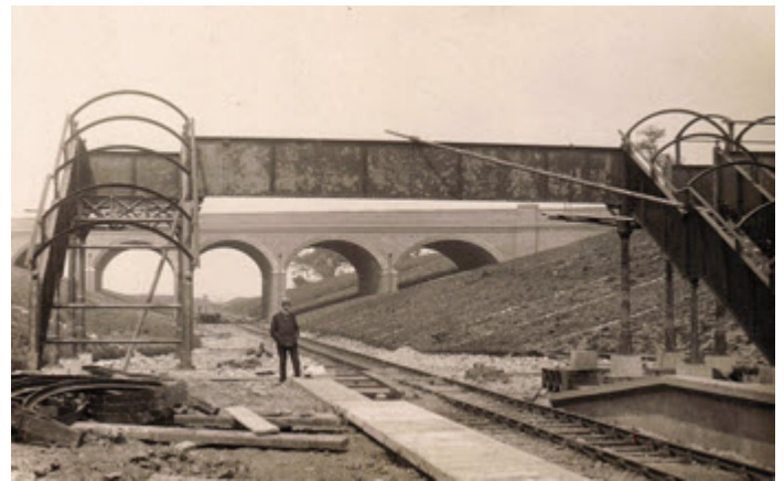
A view of Gordon Hill Station footbridge under construction in 1909 with, in the distance, the five span bridge carrying Lavender Hill across the line.
