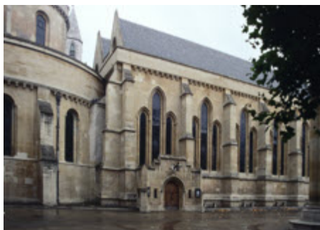
Exterior of the Temple Church, which was restored in 1825, 1841-3 and 1948-58 after extensive war damage.
