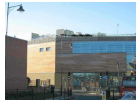
The reality - roof clutter
