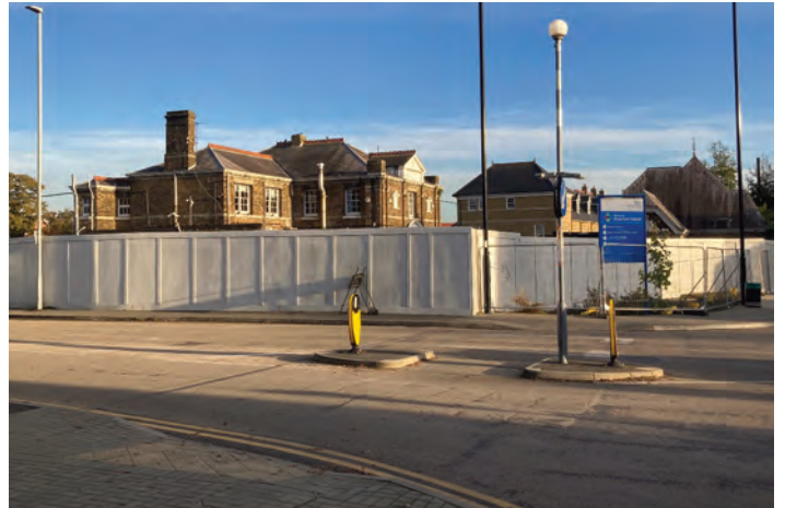
Boarded-up buildings at Chase Farm – see below
