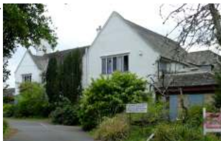
Anold House awaiting demolition
