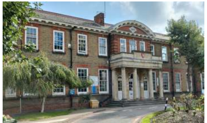
North Middlesex Hospital
