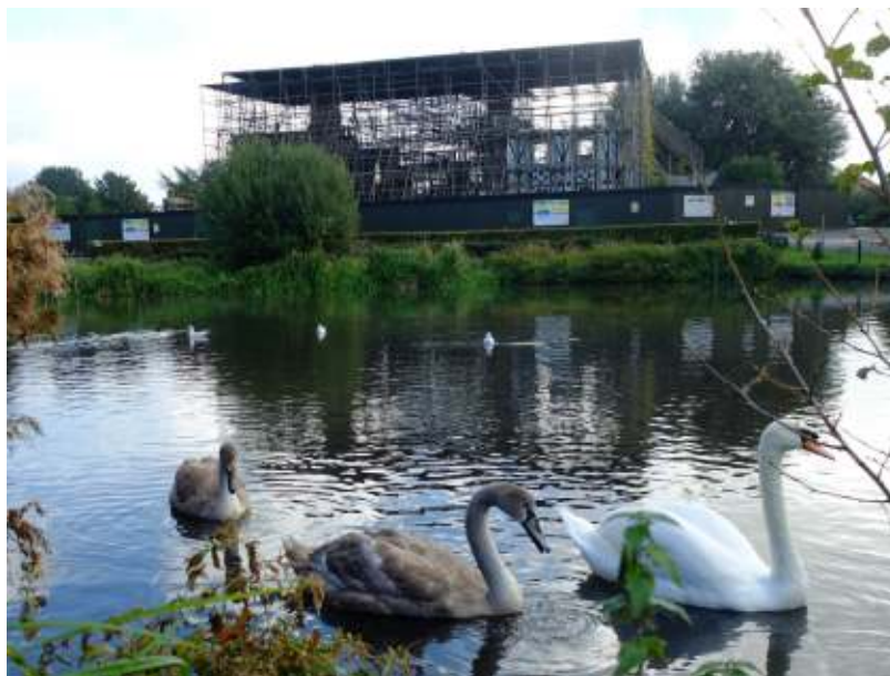
For nearly forty years the historic House has been propped up and protected by scaffolding. Is it now time to demolish the House? [Enfield Society/Andrew Lack]
