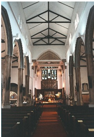
Following the discovery of dry rot in the roof in 1982, the church was closed, reopening with a new nave roof in 1985. Replacement of the side aisle roofs was completed in 1995.
