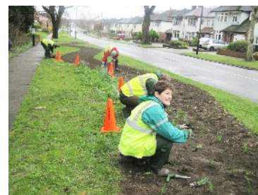
Thames21 continues to develop sustainable drainage systems (SuDS). This sinuous swale has recently been created and planted with sedges at Houndsden Road to filter road runoff.
