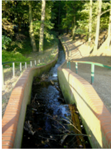
Existing spillway at Grovelands lake, to be widened to cope with floods
