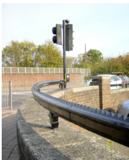
Cast iron railings at Oakwood station, in need of restoration
