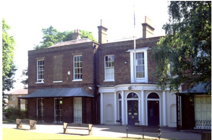
Millfield House was built by 1796 of stock brick with a stone canopied parapet. The south wing has dormer windows in a later mansard roof.
