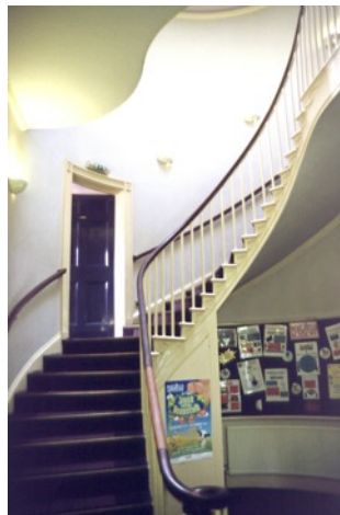
The oval stairwell has an impressive curved, cantilevered staircase, naturally lit through a glass dome. Doors and architraves are also curved to fit the shape of the wall.
