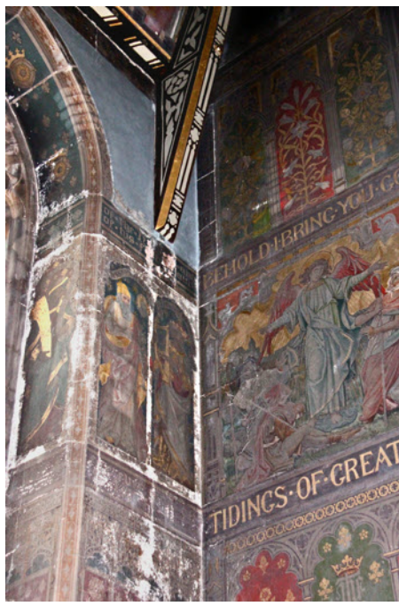
The corner of the the East Wall, showing water ingress and damage to paintings
